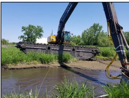
Photo of the hydraulic dredge removing legacy sediments from Dorn Creek.
