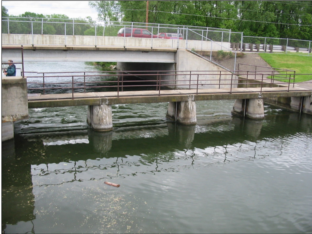
Figure 7. Dam at Babcock County Park, Outlet from Lakes Monona and Waubesa
